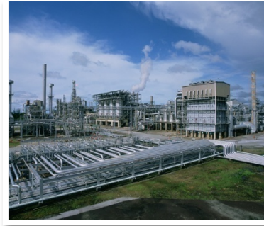
Bintulu Malaysia current capacity 14,700 bbl/d
